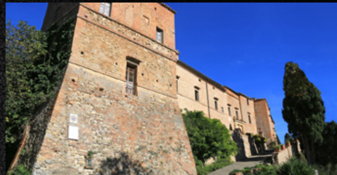
B astione e rampa d'ingresso Bastion and entrance ramp
